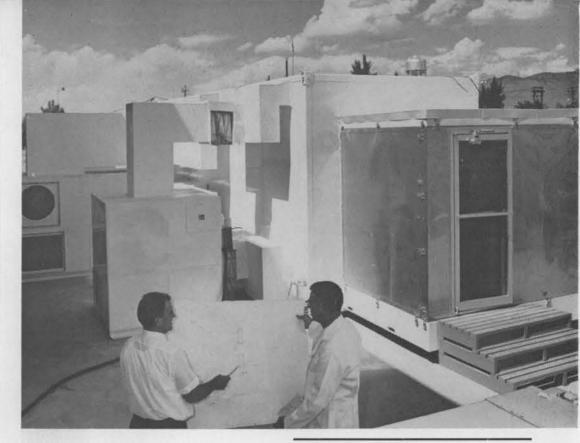
PORTABLE CLEAN ROOM is fabricated from three trailer units. Conventional components make up the air moving equipment. Willis Whitfield, left, discusses arrangement with James C. Mashburn (both 2564).
